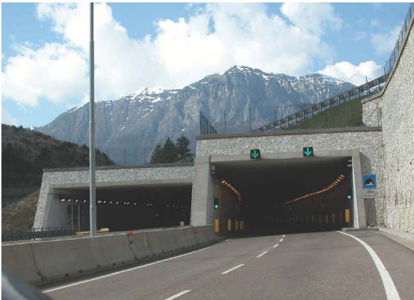
Figure 1: Tunnel deployment testbed for TRITon
